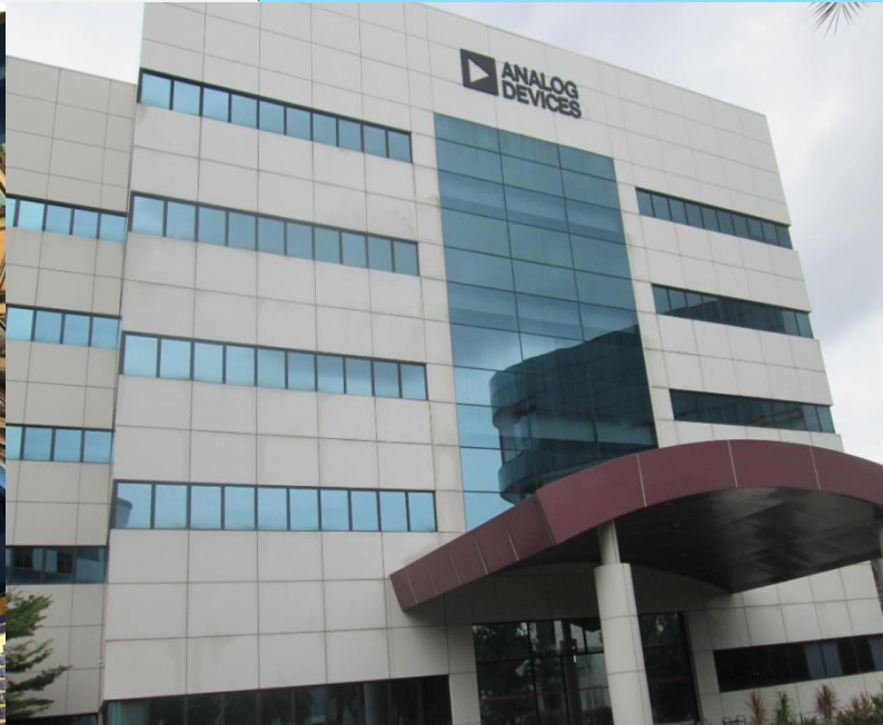
509 Yishun Industrial Park
